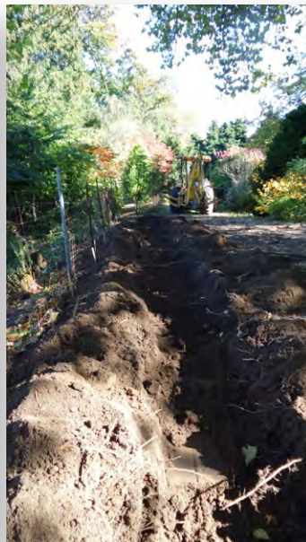
Digging the trench
